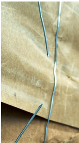
Broken strapping wires...
