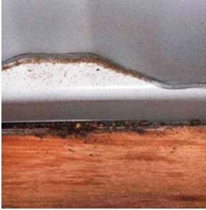
Protruding bottom side rails
