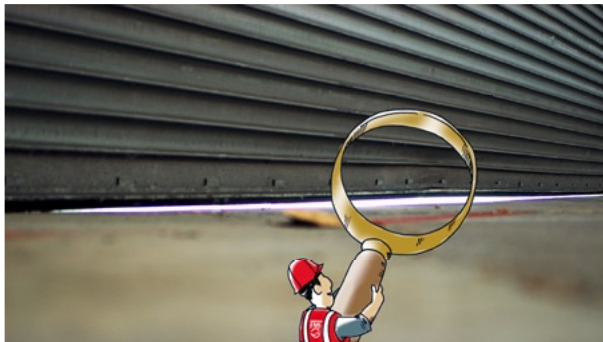
Visible space beneath rolling doors
