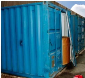
Container door damaged by cargo within
