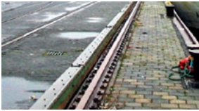
Cable duct restricts working area
